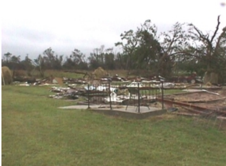
Destroyed community center building at the Green Valley Church near Dacoma in Woods County. See summary at end of May 25/26th storm reports for more information.
