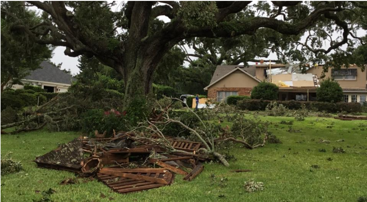
Damage to a home along Hoffner Avenue (peak winds estimated 85-90 mph, EF-1)
