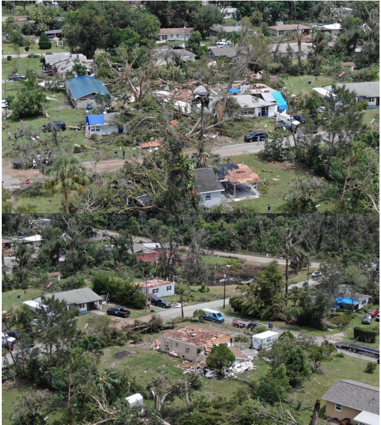
Aerial images of EF-2 damage along E Washington Ave. (source: Volusia County Emergency Management)
