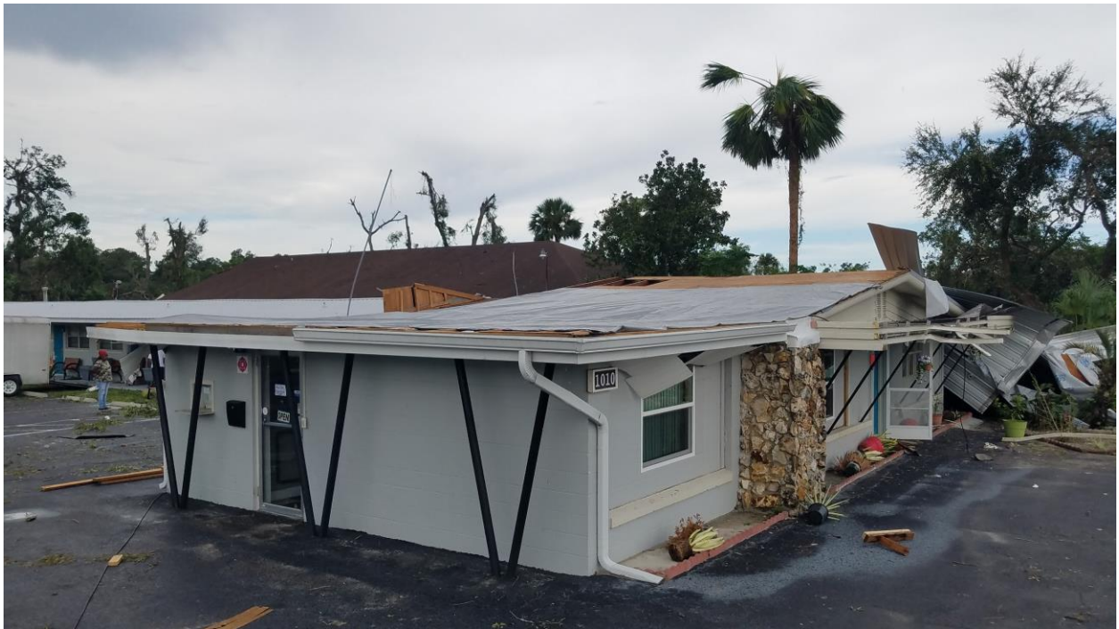
Damage to a building along North Woodland Blvd.
