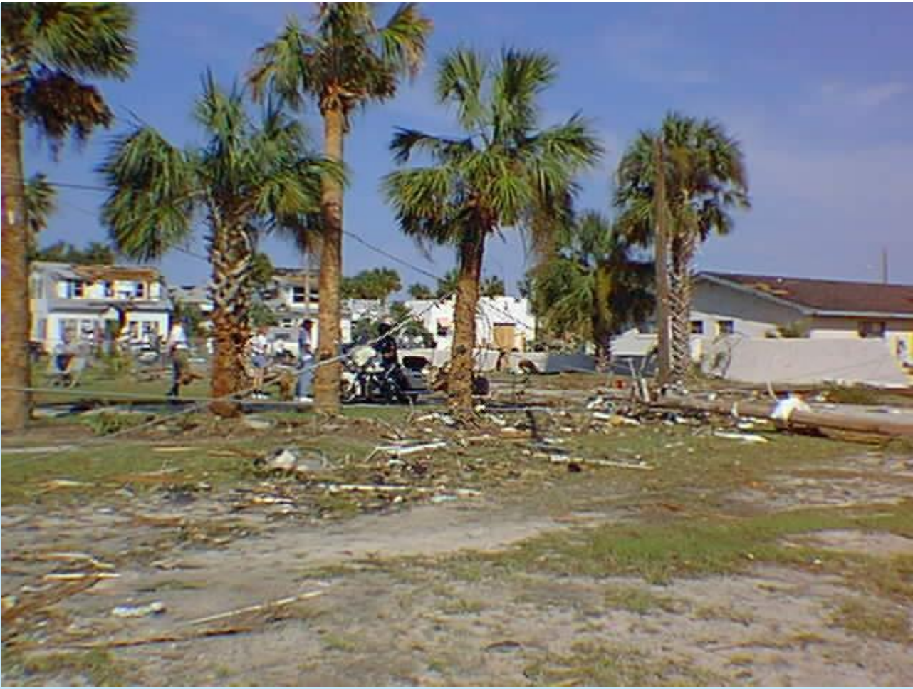
Location 3. Debris field.
