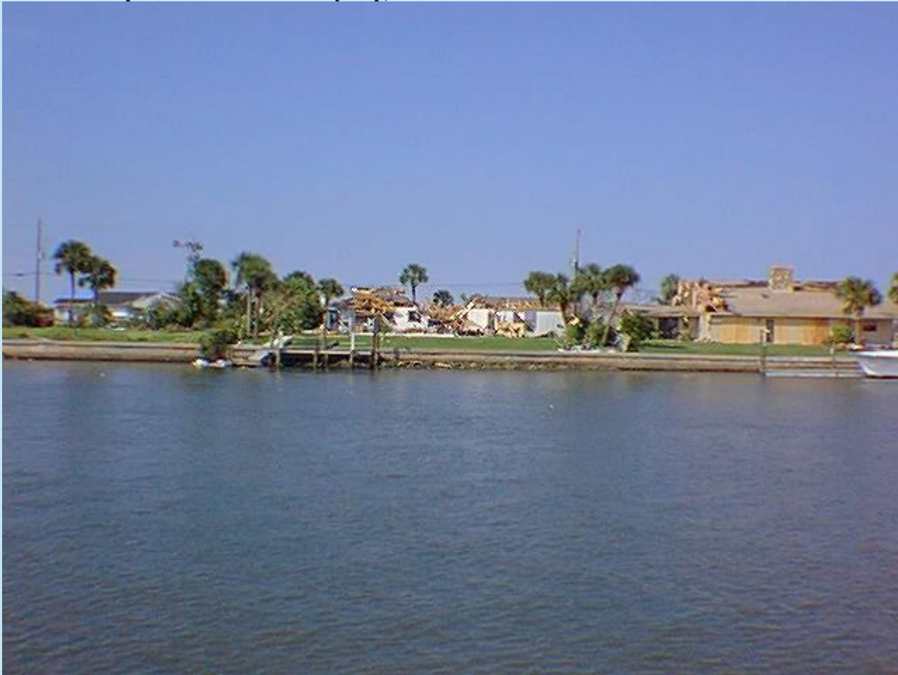
Location 1. Damage to canal
