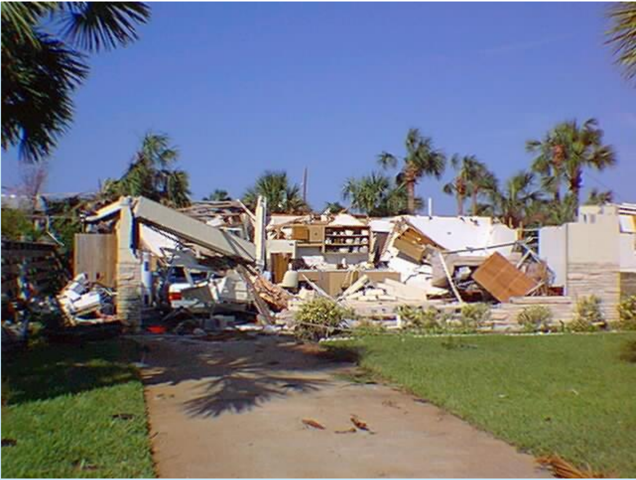
Location 4. Damage to a home.
