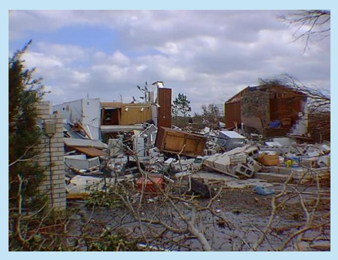
Looking through the garage door of a severely damaged concrete-block and brick veneer building.
