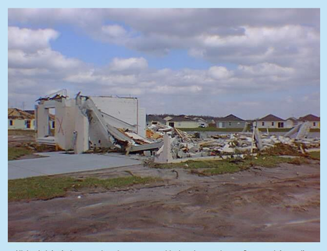
All that is left of what was a brand-new concrete-block and stucco home, Structure left standing is front-door entryway and one partial wall with a window. This subdivision was directly across the Florida Turnpike from the RV Park, where damage photos above were taken.
