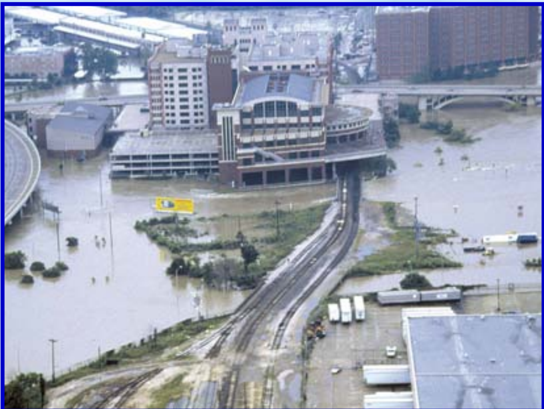
Figure 12 – Major Flooding in Houston (Courtesy of Harris County Flood Control)
