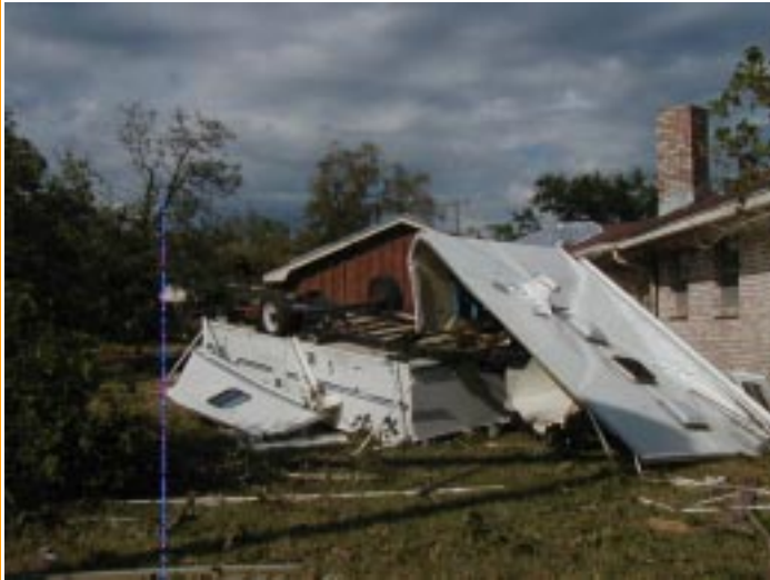
Damage done in Bryan by an F1 tornado on 10/05/03.
