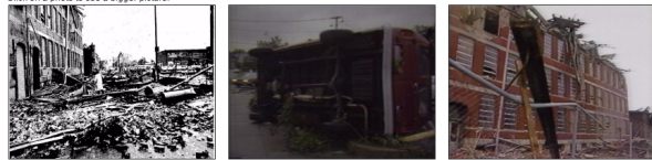
Above: A four-story jewelry manufacturing building in Providence that had its top story blown off by the tornado. Photo in NOAA Archives courtesy of the Providence Journal. Above: A truck flipped by the 1986 Cranston-Providence tornado. Picture courtesy of T.J. Del Santo and WPRI-TV. Above: Fulford Manufacturing Building after the 1986 tornado hit it. Picture courtesy of T.J. Del Santo and WPRI-TV.
